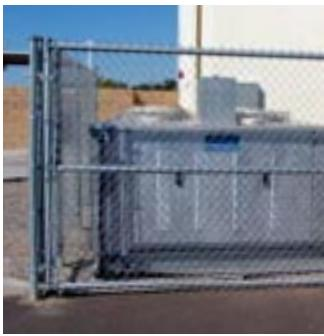
Like the rest of Tecogen's RT Series chiller line, this latest addition includes a built-in integral air-cooled condenser, which makes quick installation possible, according to Martini. The chillers' small size also allows for installation of multiple units, which gives the owner greater redundancy than is possible with a single large machine.
