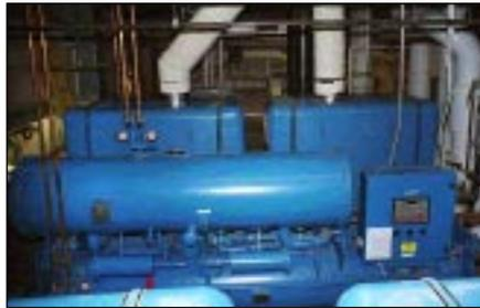
***Tecogen's first two high-efficiency TECOCHILL® DTx series water-cooled chillers, installed in a hybrid plant at Northern Westchester Hospital Center, Mount Kisco, N.Y., helped the hospital realize a beneficial cooling season.***
