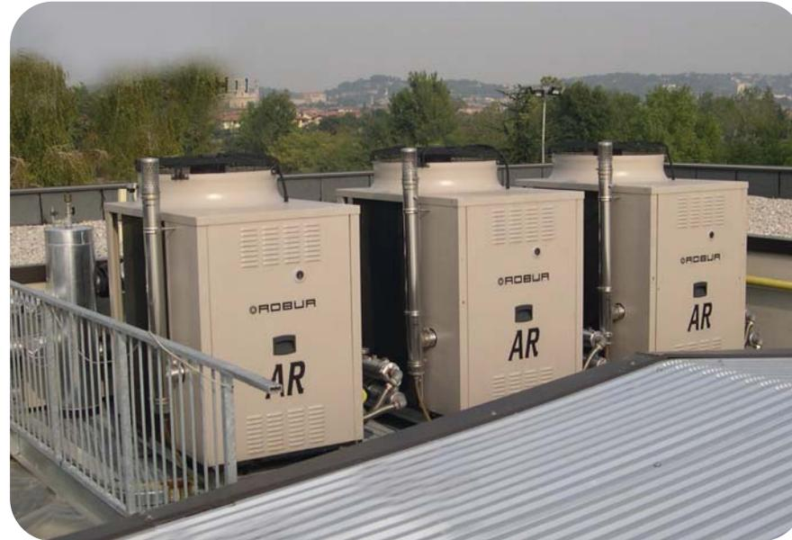
Evaluation of the capability of the heat exchange surface has been carried out, since heat pump operating temperatures are typically lower than those of traditional boilers and fan coils size turned out to be adequate for the system load. **Thus, no change to the whole indoor plant was required.**
