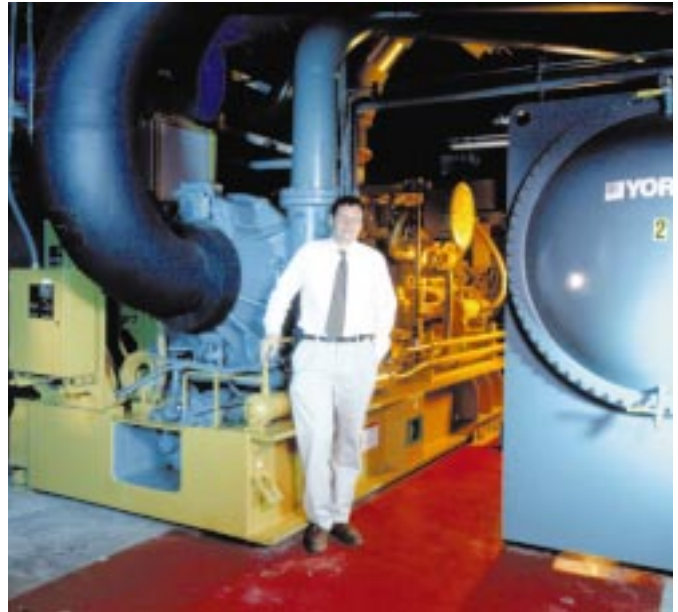
(upper left) – The hybrid cooling plant features an 1,800-ton YORK Millennium YG natural-gas-engine-drive chiller and two 1,500-ton YORK electric-drive centrifugal chillers.
