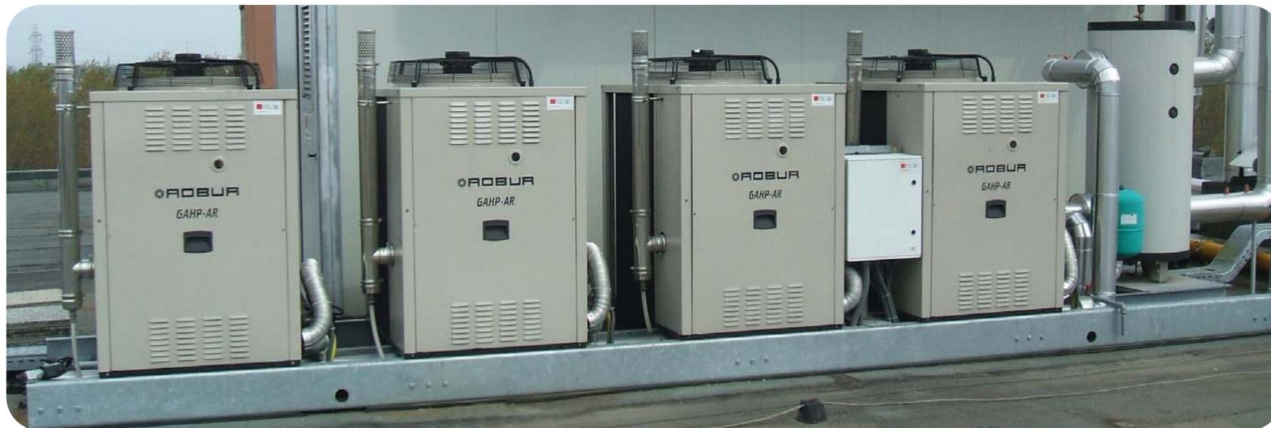
Thanks to modularity of the Robur system, the design engineer chose 5 GAHP RTAR240-480 units. The inlet water temperature is 113 °F during winter season and 55.4 °F during summer season. The design planned a wall air conditioning system integrated with a primary air system for air replacement and dehumidification during summer season. The wall embedded (composed by 0.4-inches polypropylene
