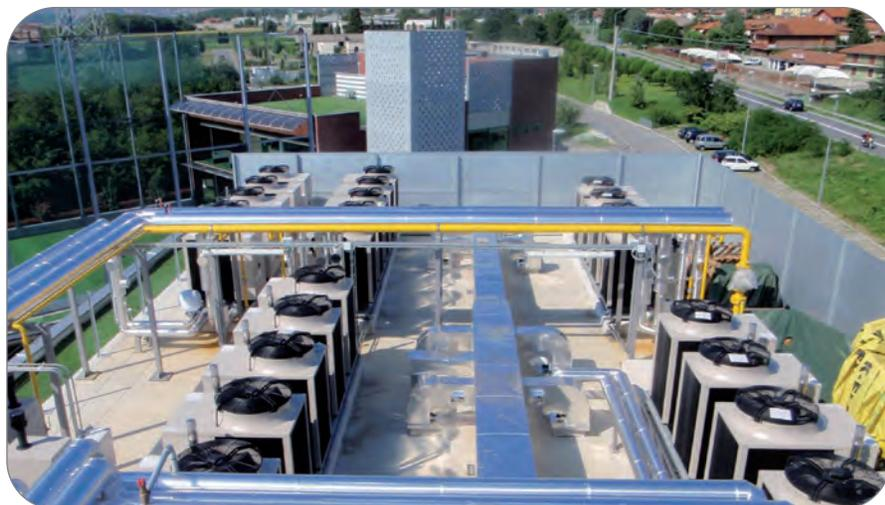
of DHW and 1,387,000 Btu/h (115.5 tons) cooling capacity. Overall requirements are satisfied by five preassembled gas-fired absorption links with reversible cycle heat pumps, chillers for cooling and chillers with heat recovery. The links have been installed on the roof, thus saving space.
