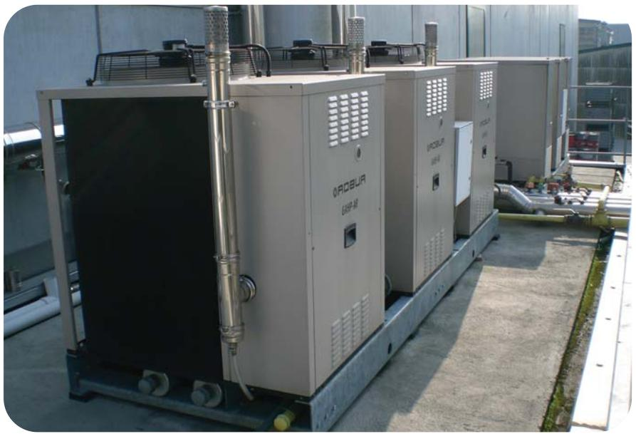
The Robur Gas Absorption Heat Pumps provide very high heating efficiency, thanks to ammonia that recovers thermal energy also at very low ambient temperatures.
