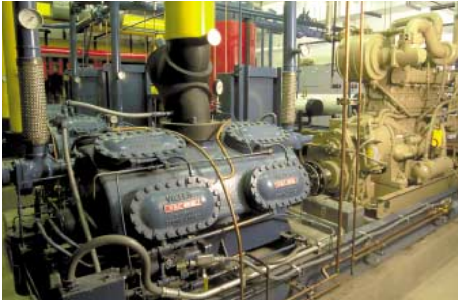
A 350-horsepower Cummins natural gas engine-driven chiller with 160-ton Vilter compressor are key components of a hybrid ice-making system at the Super Rink.
