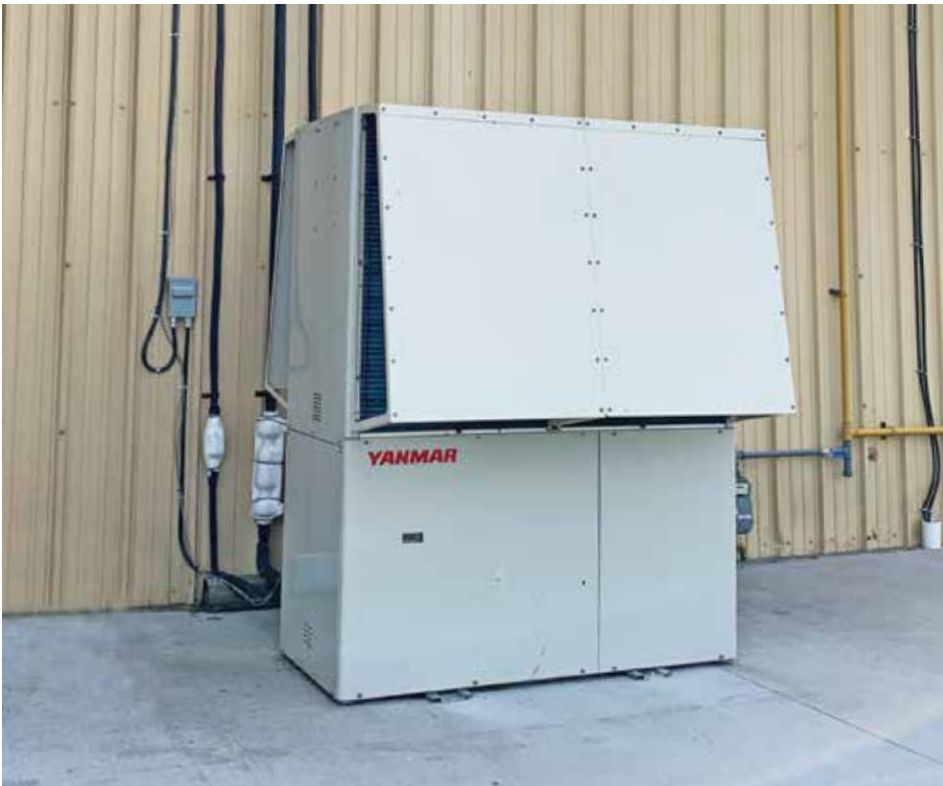
Yanmar’s Gas Heat Pump Variable Refrigerant Flow system provides both heating and cooling for Burnham Family Farm Market, which includes a bakery and a retail store.
