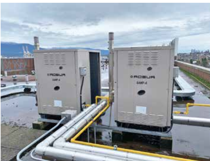
These Robur gas heat pumps have been installed at a housing complex in Vancouver, Canada, as part of a FortisBC pilot project to demonstrate that GHPs provide more than 100% efficiency, lower emissions and reduce energy bills.
